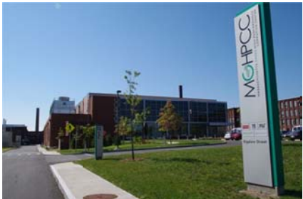
Cover photo: The Massachusetts Green High Performance Computing Center (MGHPCC), Holyoke, MA. The data center is dedicated to supporting the growing research computing needs of five of the most research-intensive universities in Massachusetts: Boston University (BU), Harvard University, MIT, Northeastern University, and the University of Massachusetts (UMass). Photo by Joseph Bednar, Businesswest.
